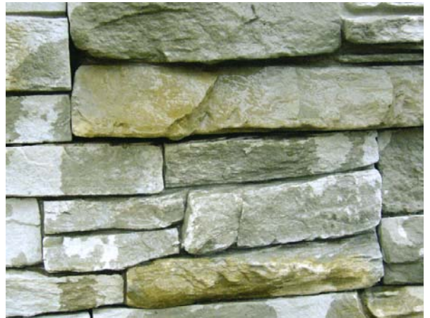
▲矽封劑 SE-2025 施工前(Before treatment)
