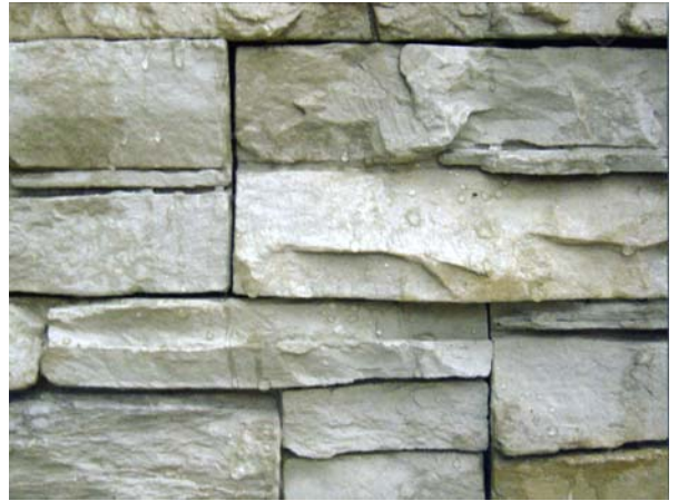
▲矽封劑 SE-2025 施工後(After treatment)
