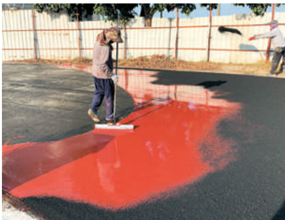
PU基層施作(含複合顆粒) PU base layer (with composite granules)
