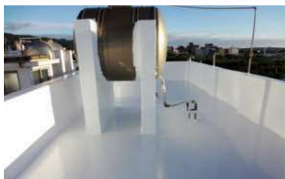
PU防水防熱型 Waterproofing and Heat-proofing
