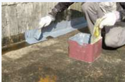
牆角補強施工 Reinforcement at corners
