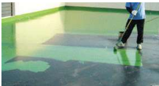
面漆塗佈 Top coating
