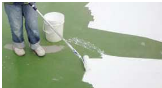
防熱塗佈 Heat-resistance material spread
