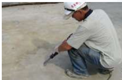
剷除凸出物、雜物 Eliminate all the contamination
