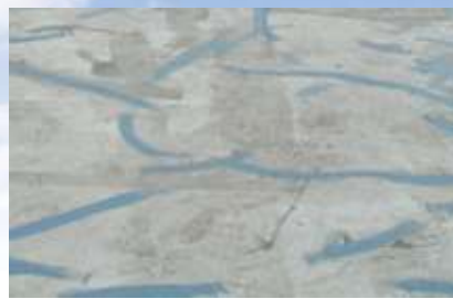
地板裂縫補強施工 Reinforcement at cracks
